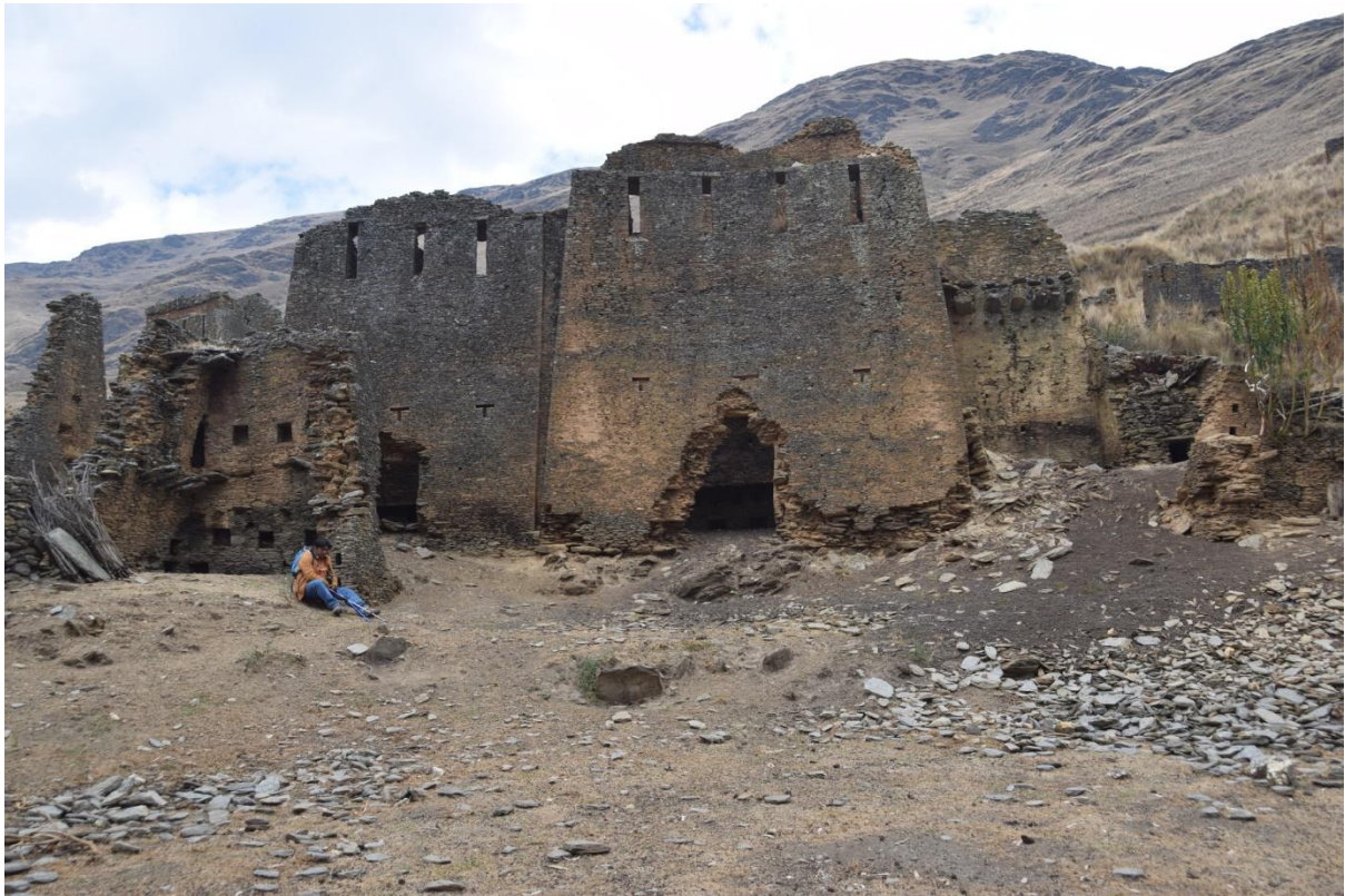
Front of a complex of three large torreones side by side. Note: only the rear and parts of the side walls remain of the torreón on the right hand side. There is a further, free-standing tower in front of the complex, to the far left of the picture (behind the seated person).
