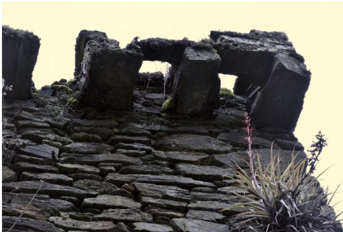
Support for the parapet at the top of the tower
