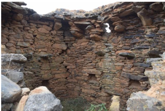
Remains of corbels over windows inside a chullpa
