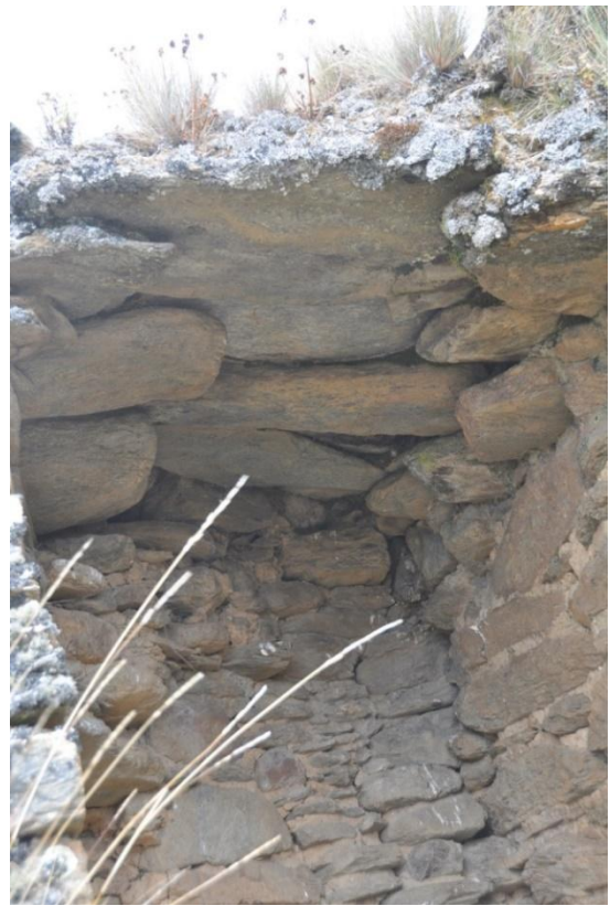
Chamber with remains of corbelled roof
