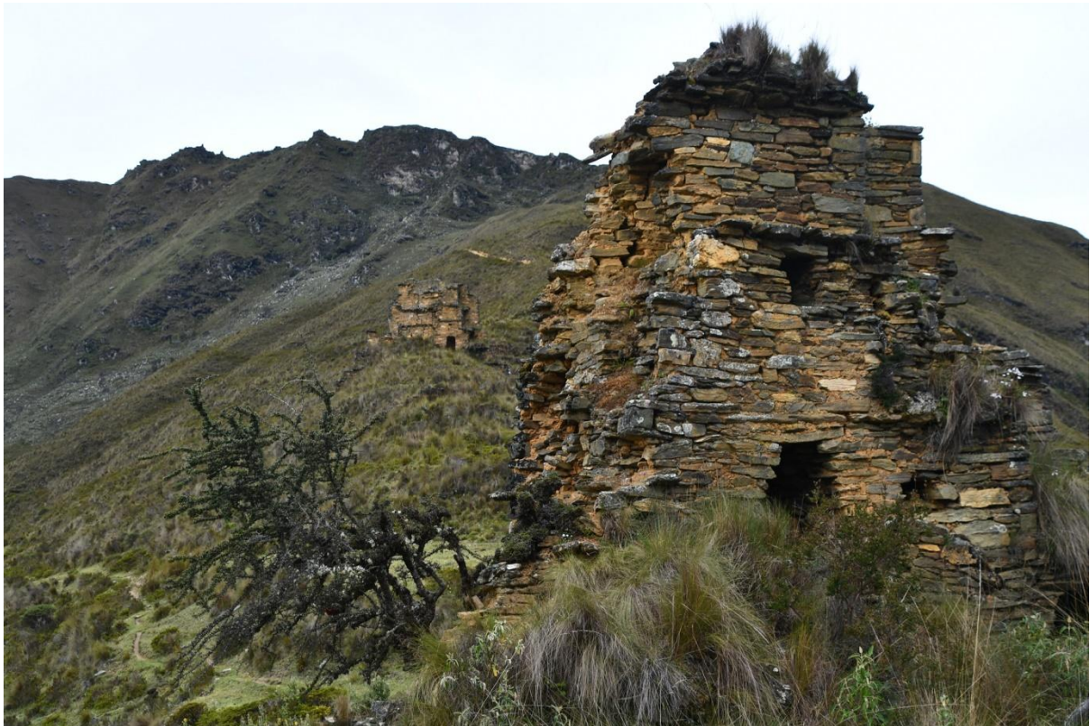
The interior faces of two headwalls, the nearer one partially collapsed. Note Auga Punta on the ridge line at top left.
