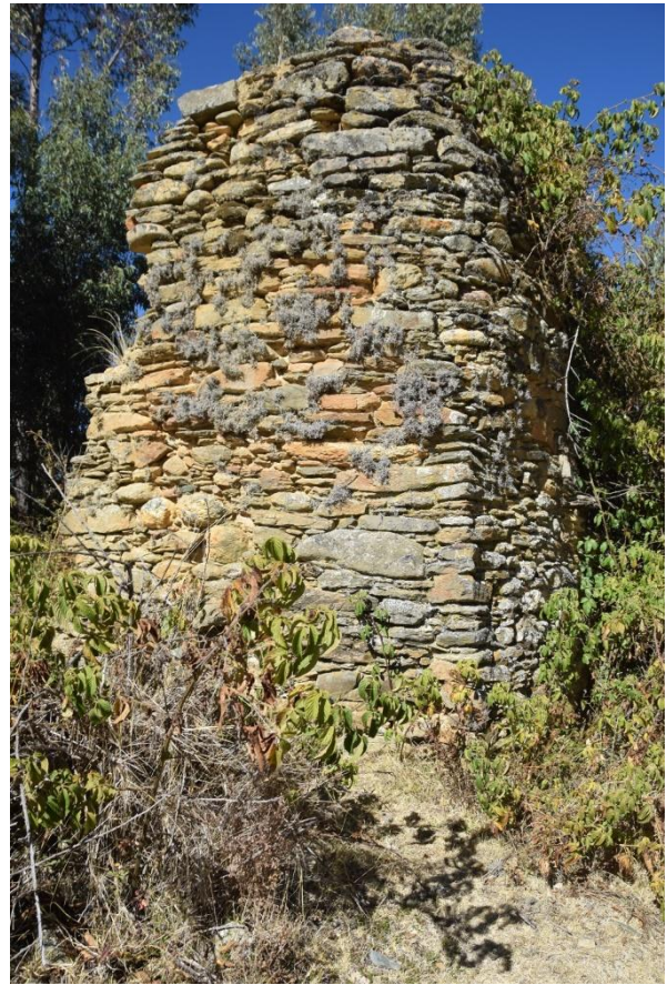
Corbel vaulted tower structures
