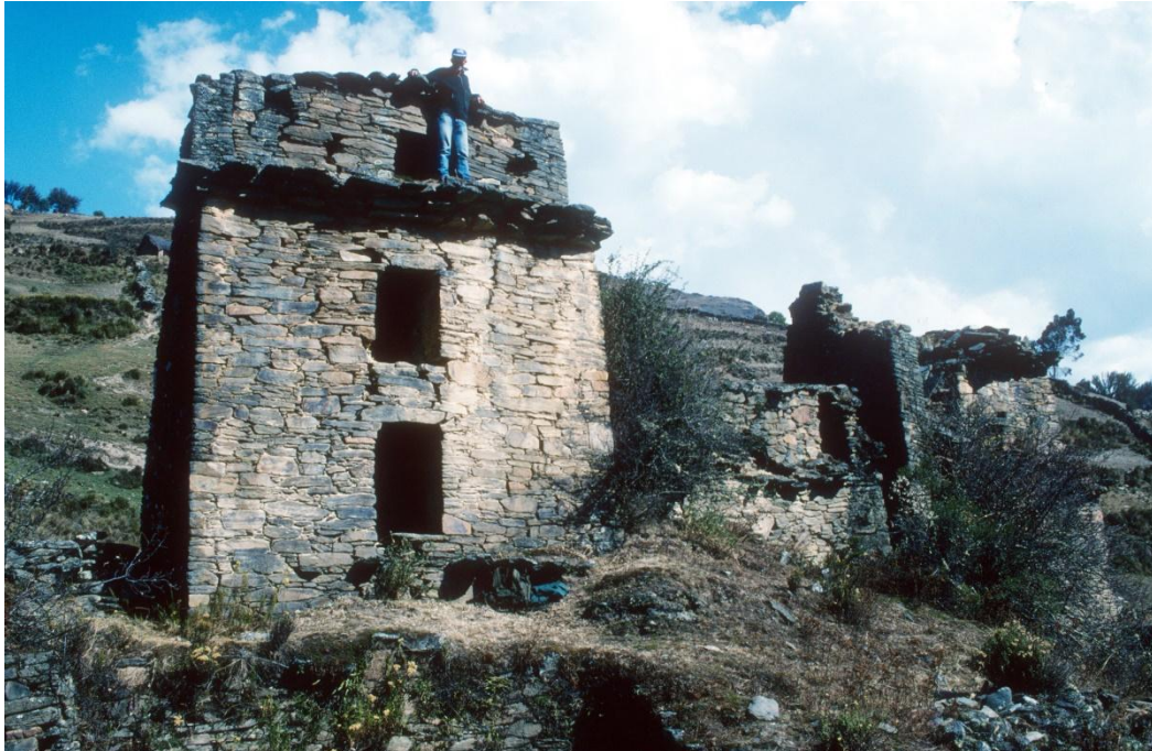
Interior side of a headwall (1996)
