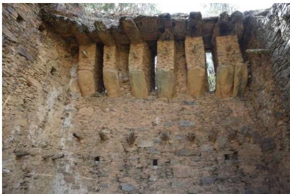
Detail of corbel vaulting of a torreón
