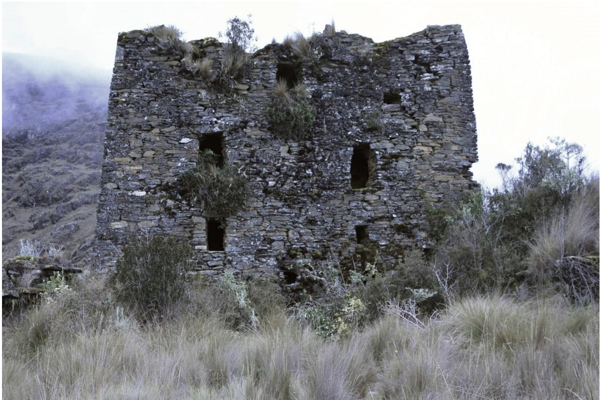
Interior side of the headwall at Tucu Waganan
