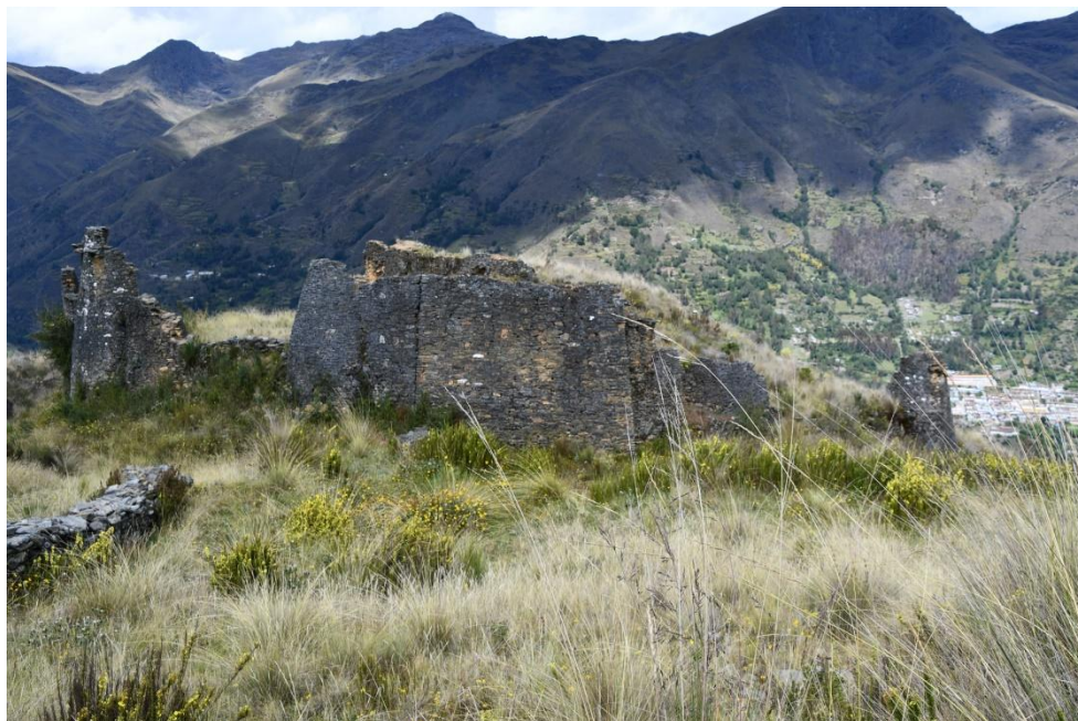
The exterior of the headwall
