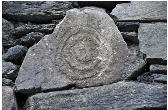
Incised stones inserted in the exterior wall
