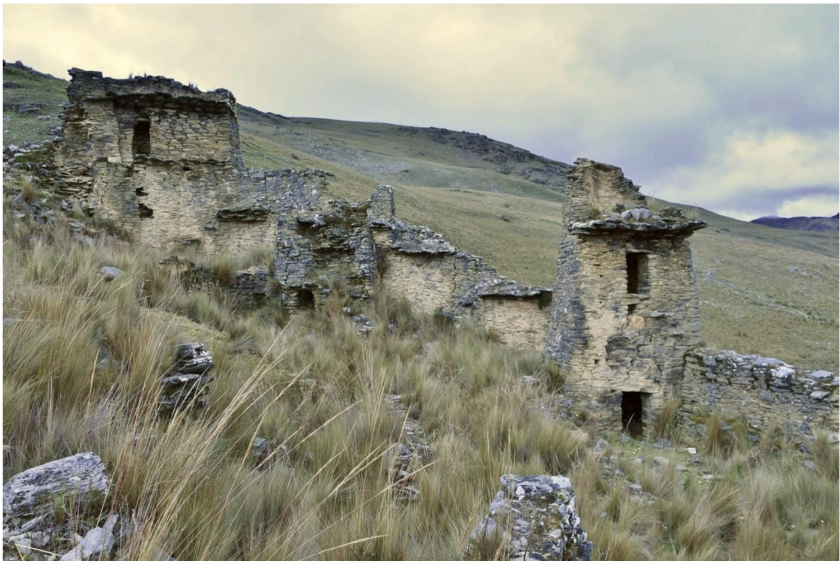
Curtain wall and tower – south side
