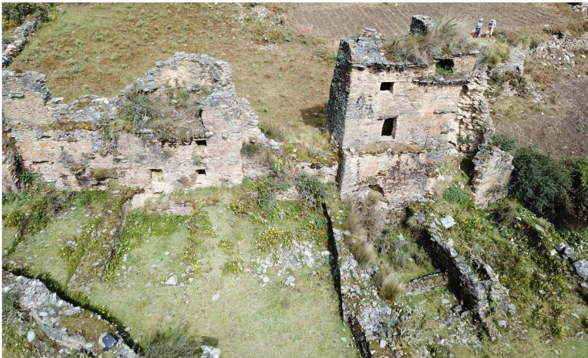
Aerial views of the site and interior sides of the headwalls
