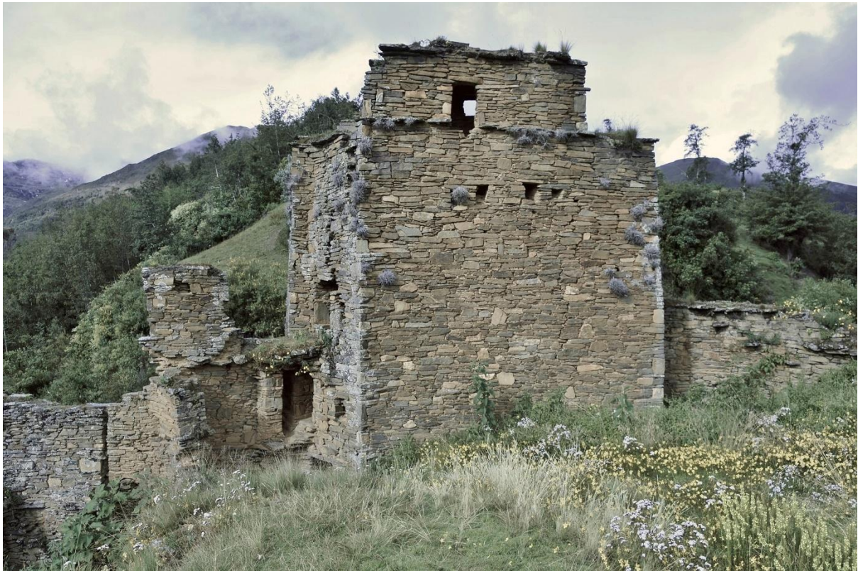
Interior side of headwall
