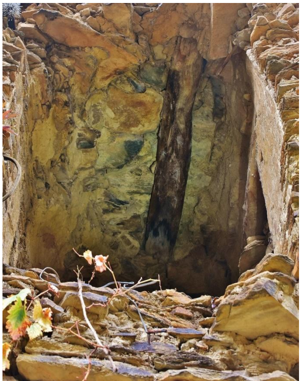
Wooden beams supporting the ceiling of the middle floor chamber
