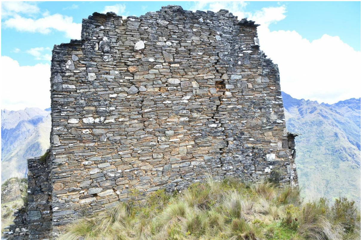
Exterior of the headwall in the background of the picture at the top of the page. Note the engraved stones part way up the wall. For details see the previous page.
