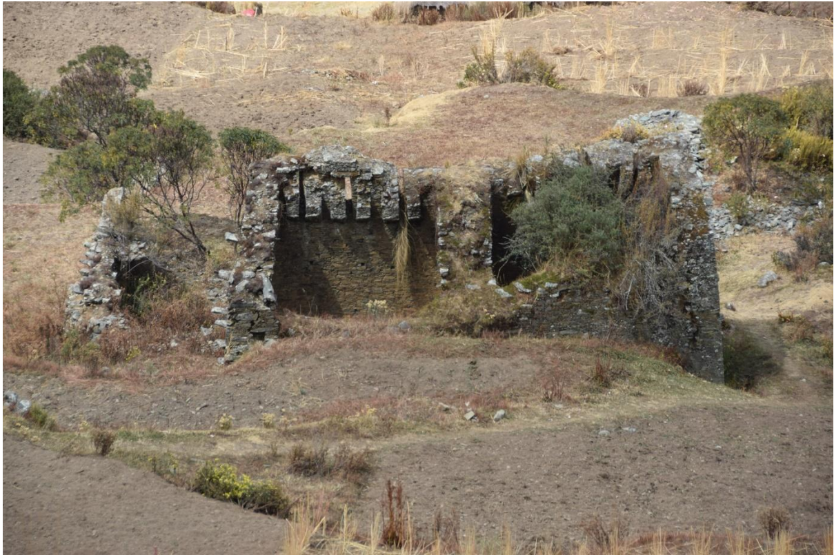
A tree growing out of a tower wall at Sahuay (Chupan)
