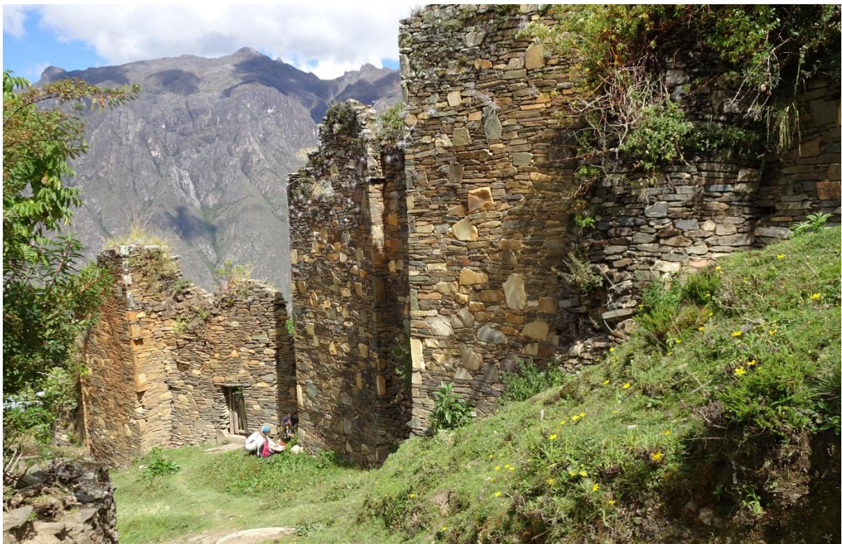
Exterior of the curtain wall south of the headwall
