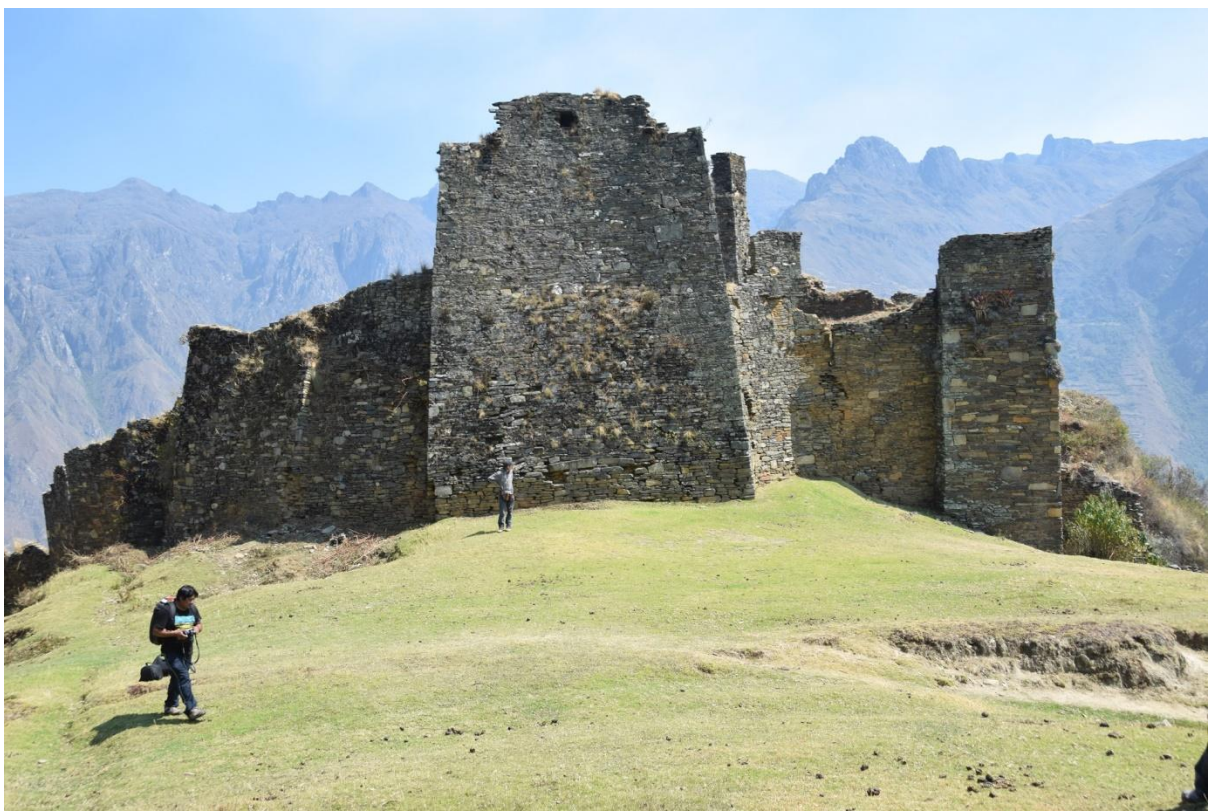
Exterior of the headwall, with part of the curtain wall to the south (at left)
