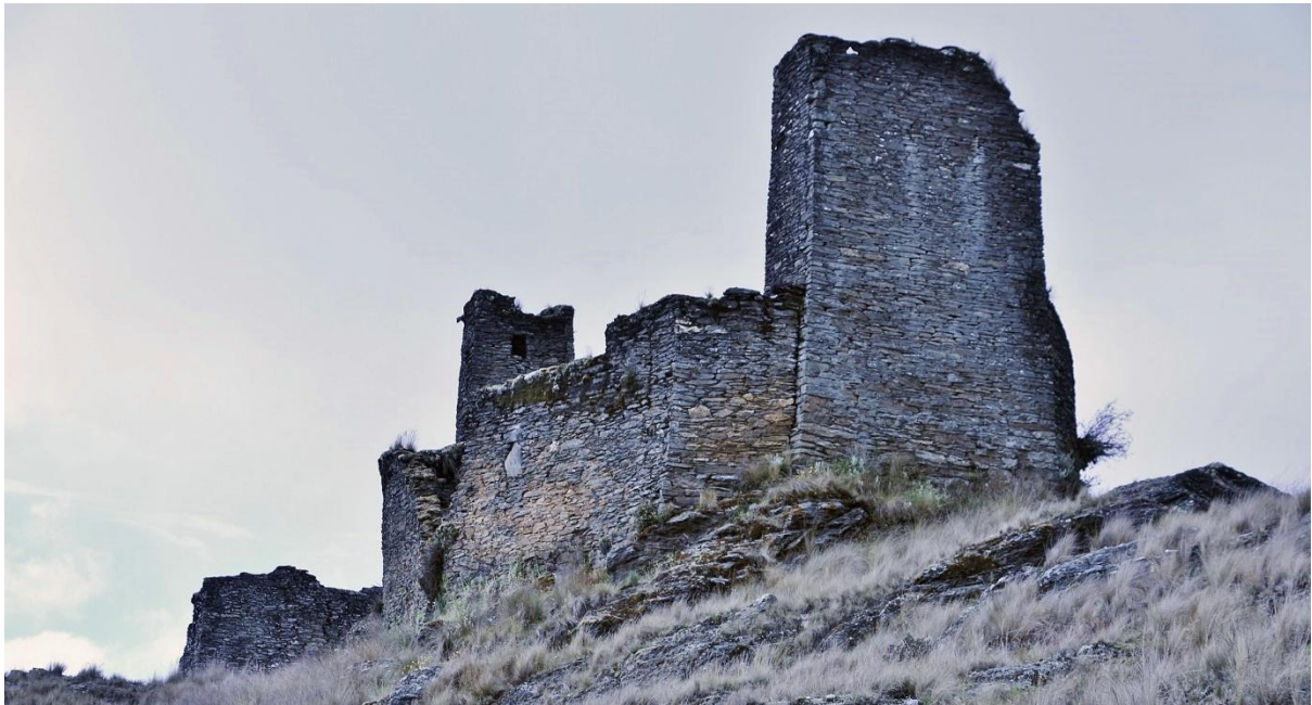
Exterior view of the site from the headwall end (facing south-east)
