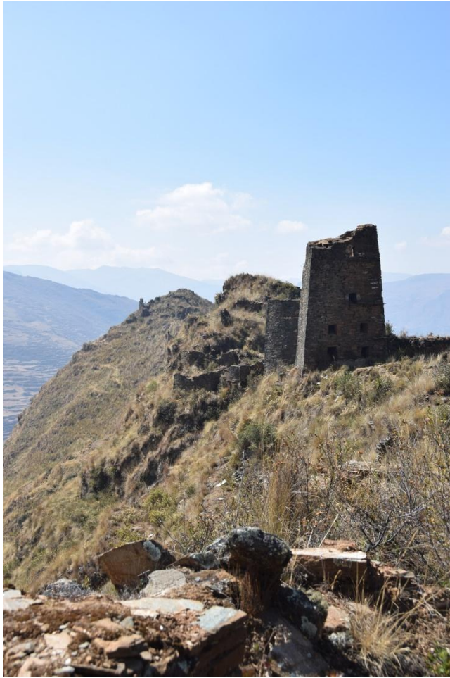
View along the ridge, facing east
