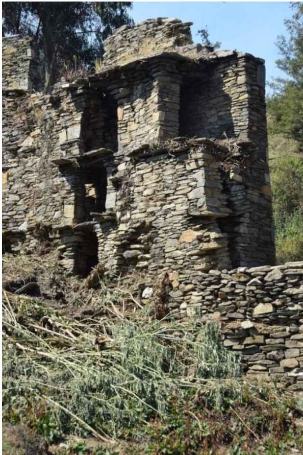
Detail of interior of the curtain wall
