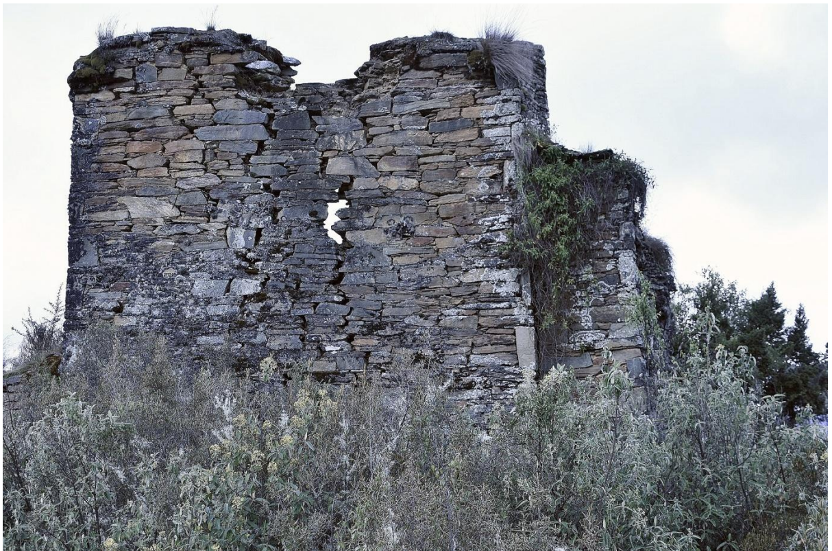
Exterior of the headwall
