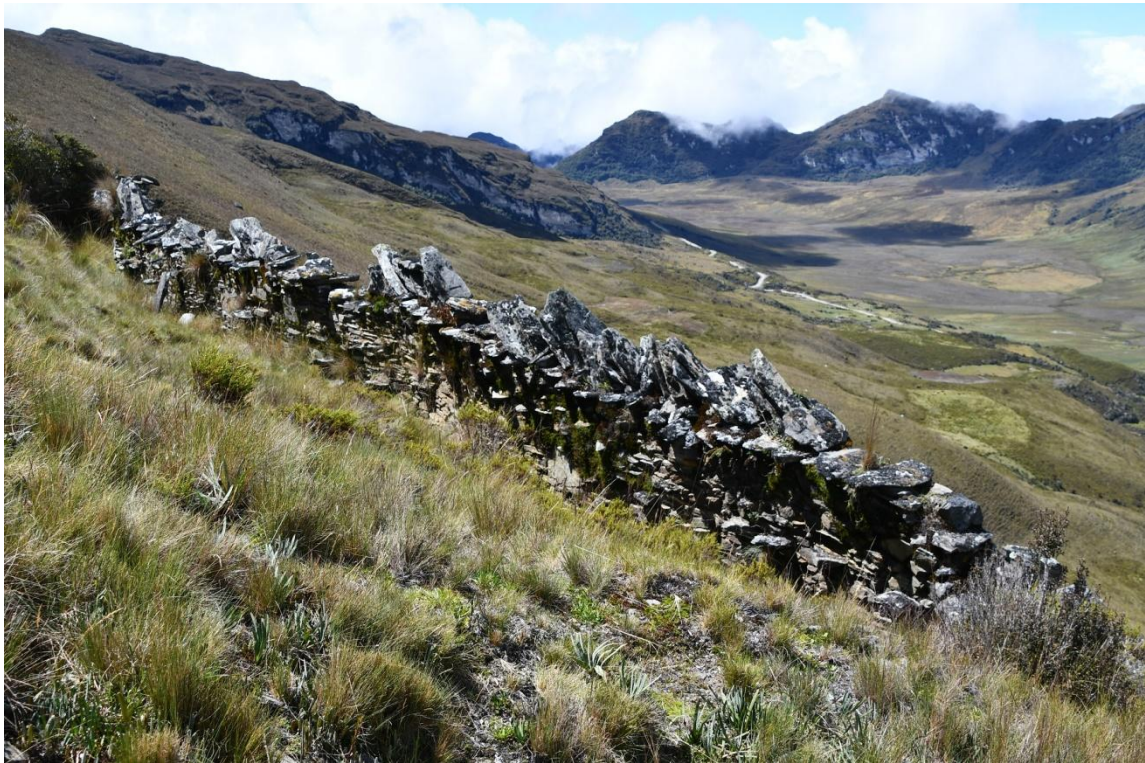
Section of the outer curtain wall on the south side of the complex. The road to Monzón is in the distance.
