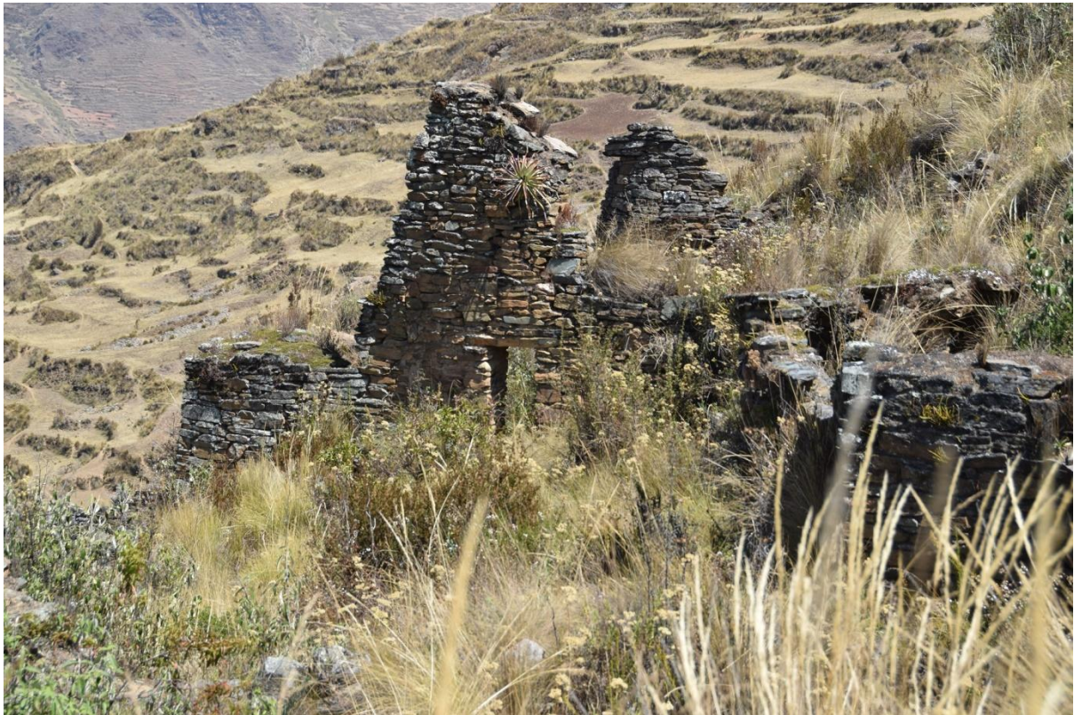
Inca period structure. Note the gable wall.
