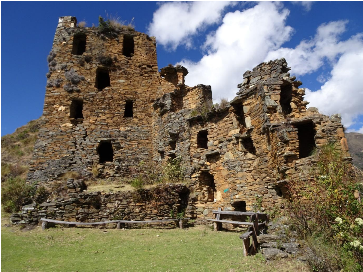
Interior side of the headwall at the bottom of the site
