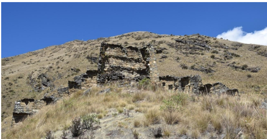
Inner side of the headwall with flanking defensive walls. The front wall has fallen away, revealing the galleries within the headwall.
