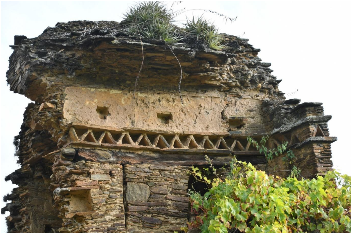
Exterior wall of the upper chamber, facing the open platform. Note the Andean crosses in the adobe plastered wall above the Chachapoyas style zigzag decoration and the wooden beam immediately below that decoration.
