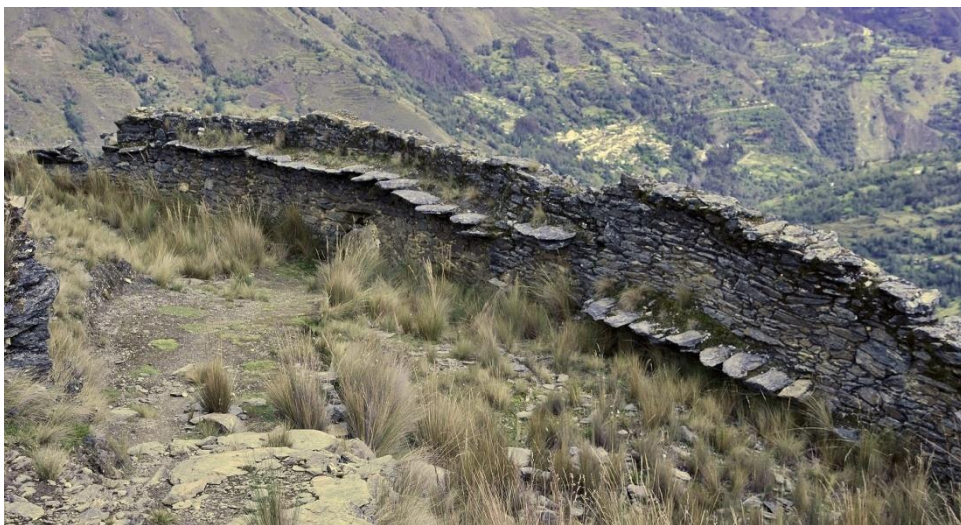
Interior of the curtain wall, with walkway on the inner side
