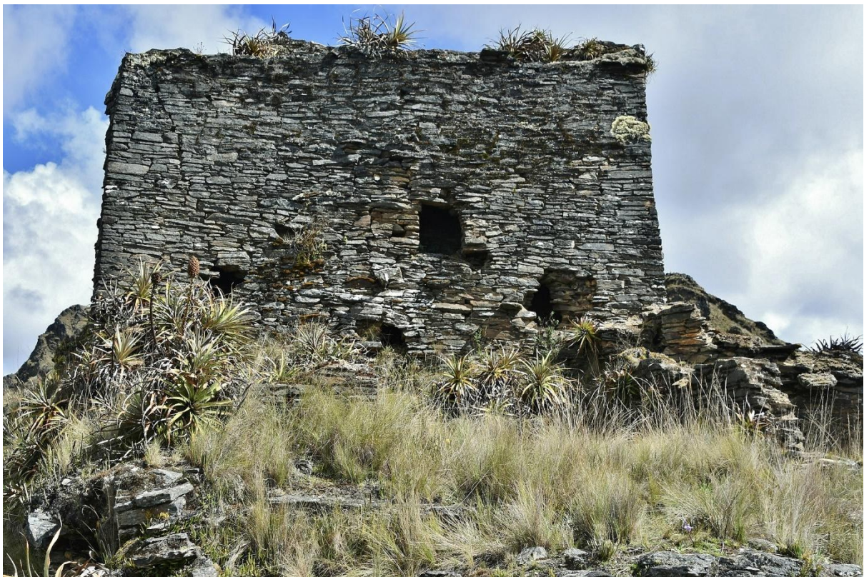
The building with the white band of quartz, north face. Note: no white quartz this side.
