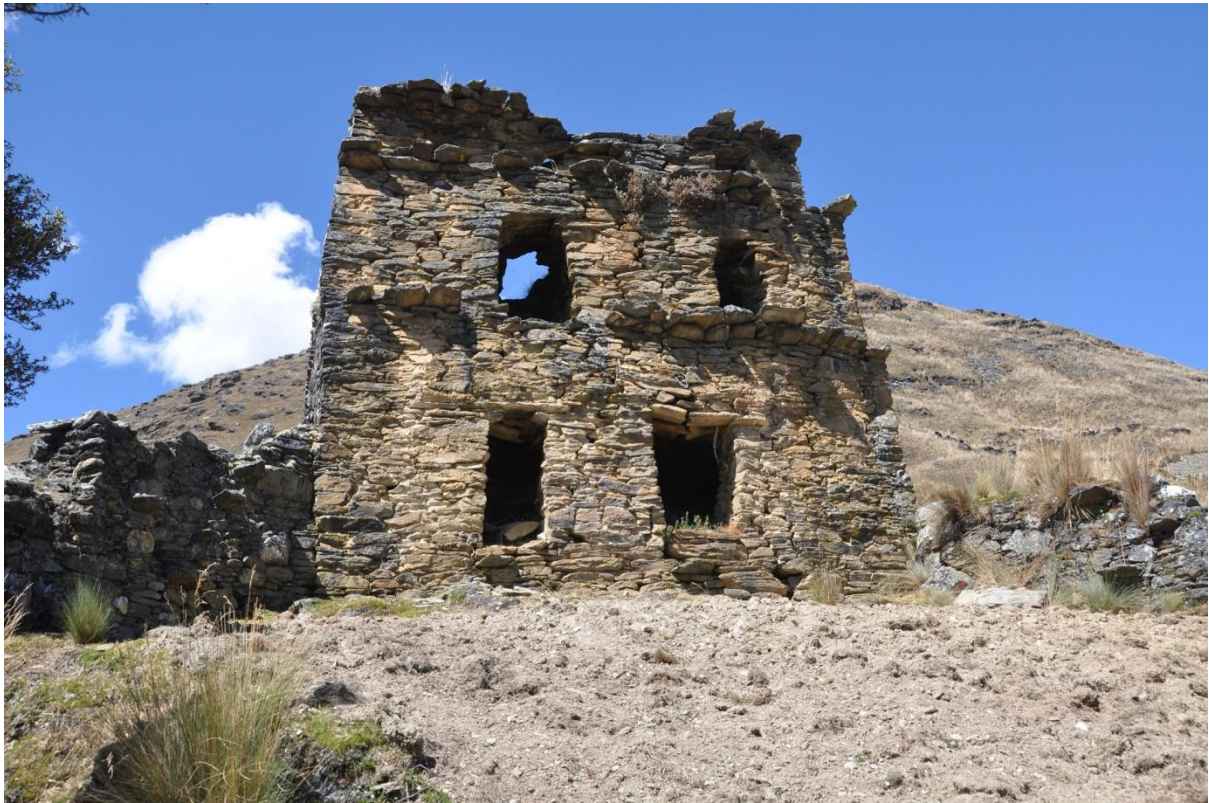
The inner side of the headwall
