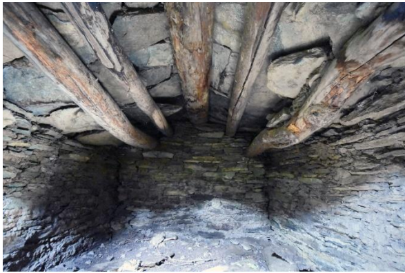
Wooden beams supporting the roof
