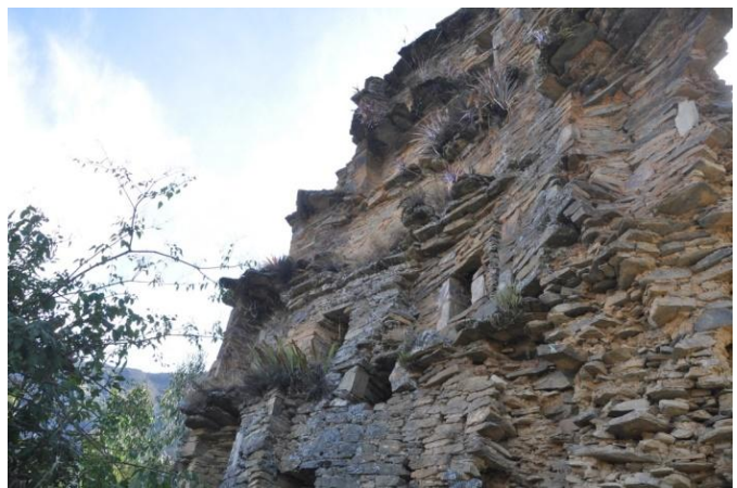
The interior side of the headwall, which has collapsed higher up
