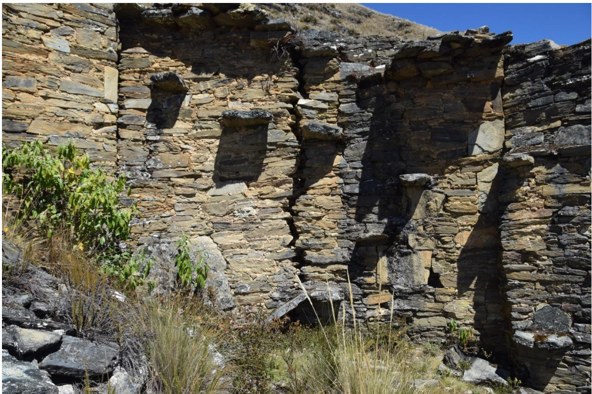
Interior of part of the defensive curtain wall. Note the steps jutting out of the wall.
