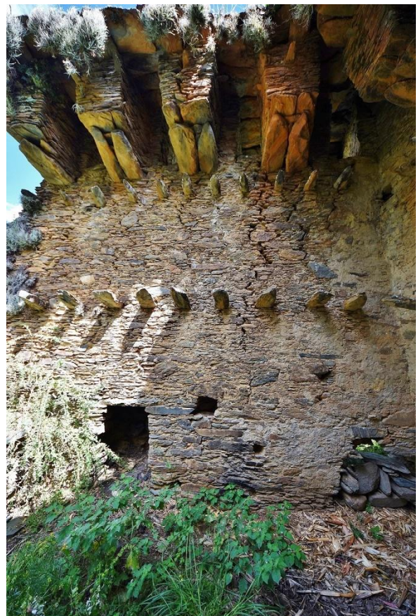
Interior of a torreón, with details of the corbel vaulting
