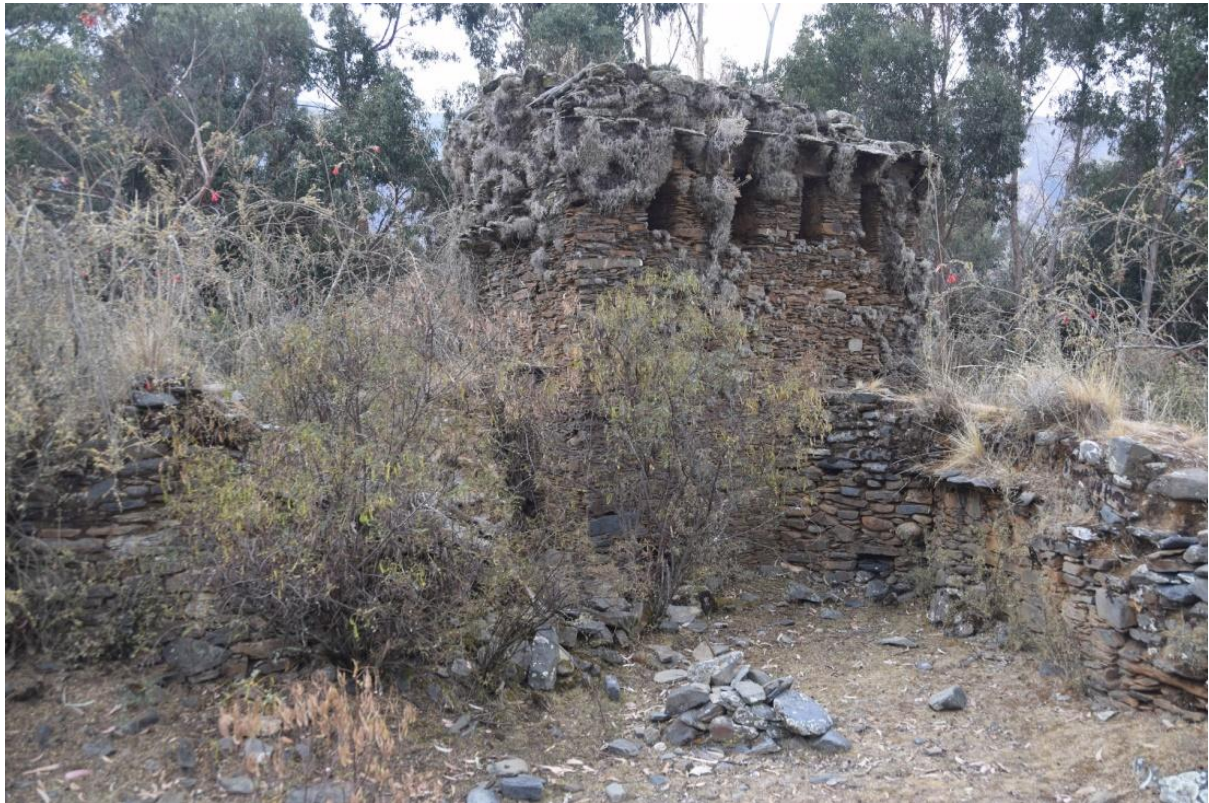
Exterior remains of a torreón. Note the characteristic upper windows.
