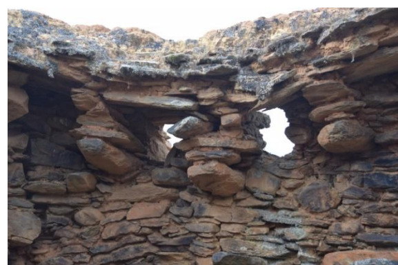
Remains of corbels over windows inside a chullpa
