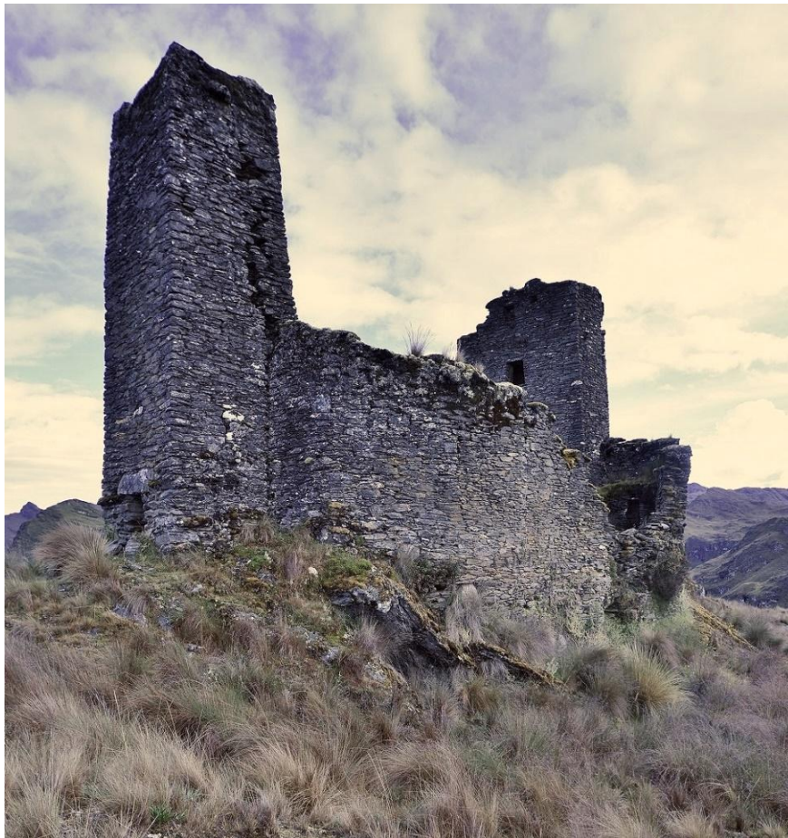
Exterior view of the site from the entrance tower end (facing south-west)
