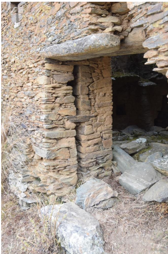
Detail of the double wall construction of a doorway jamb, common in torreones
