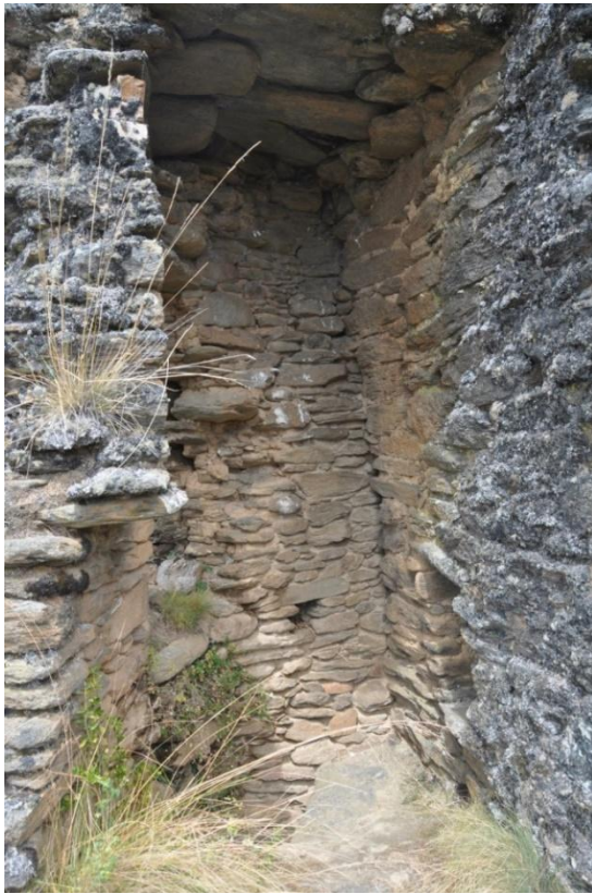
Chamber with remains of corbelled roof
