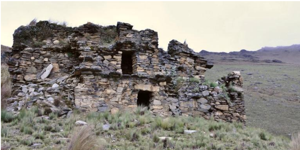
Lower right structure: probably a headwall (1996 above, 2017 below). Note how the left front section of the wall has fallen away since 1996.
