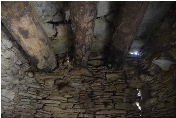
Wooden beams supporting the ceiling of the middle floor chamber
