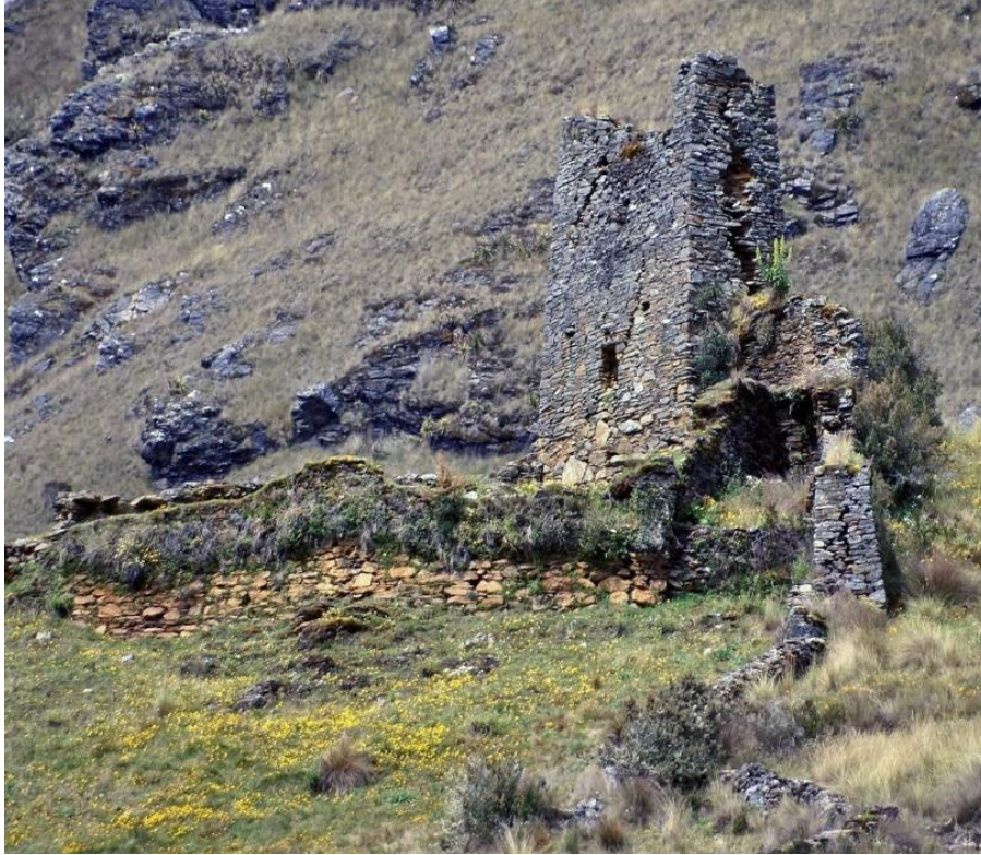
Side of the headwall facing into the settlement, with remains of the curtain wall
