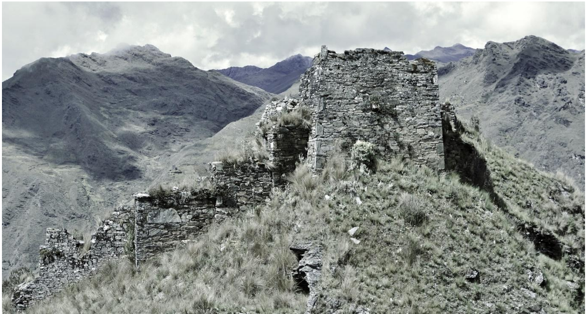
Exterior view of the headwall of Purwa Castillo and part of the curtain wall
