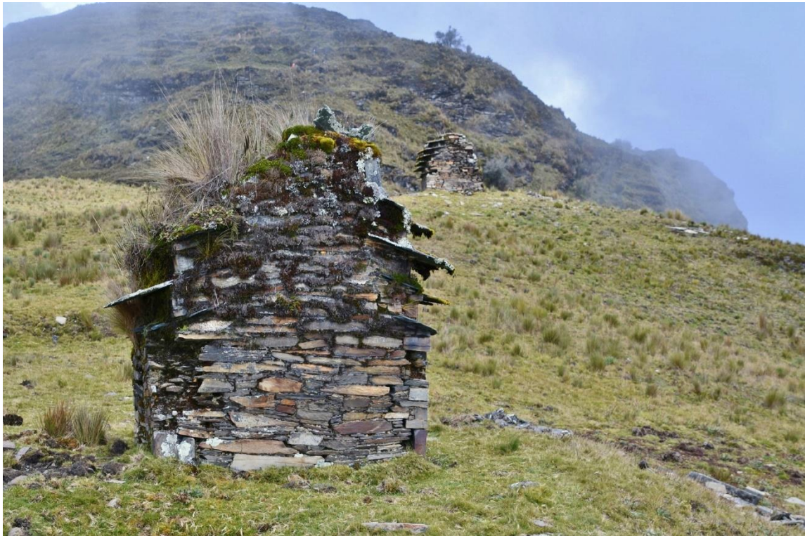
This is charnel house No. 2, with No. 3 in the background and the hill with ruins beyond
