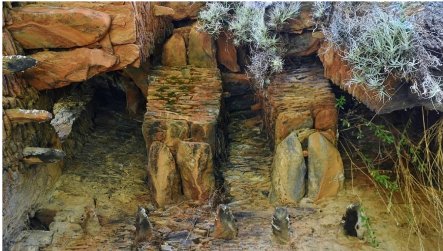
Corbels at the junction of the end and side walls
