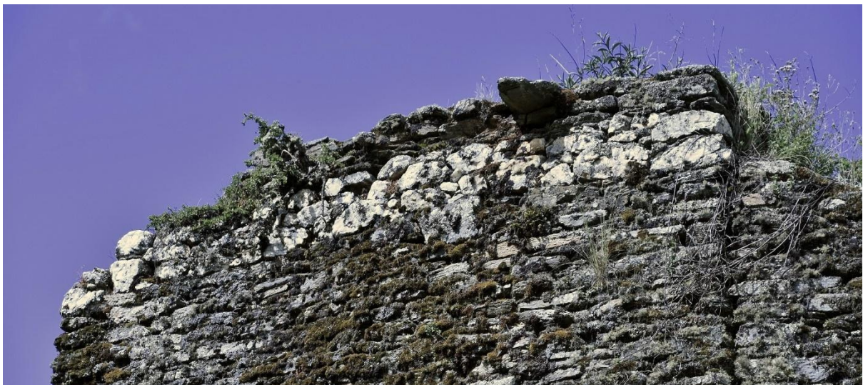
Top of the exterior of the headwall. Note the band of white quartz.
