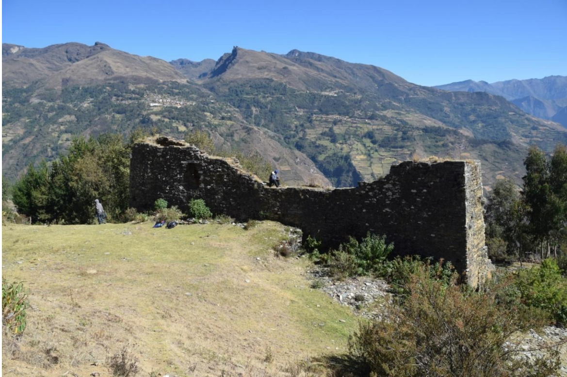
Rear of the headwall and view to the north-west
