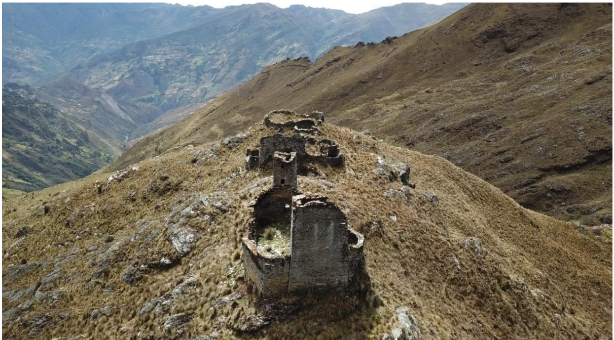
Aerial view of the site. Headwall in the foreground. Other structures beyond.
