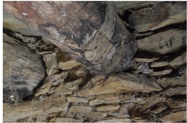
Wooden beams supporting the ceiling of the middle floor chamber
