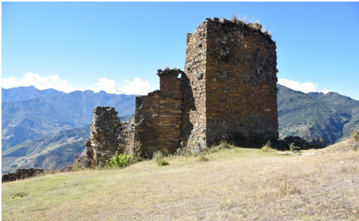
Headwall exterior, at the bottom of the site
