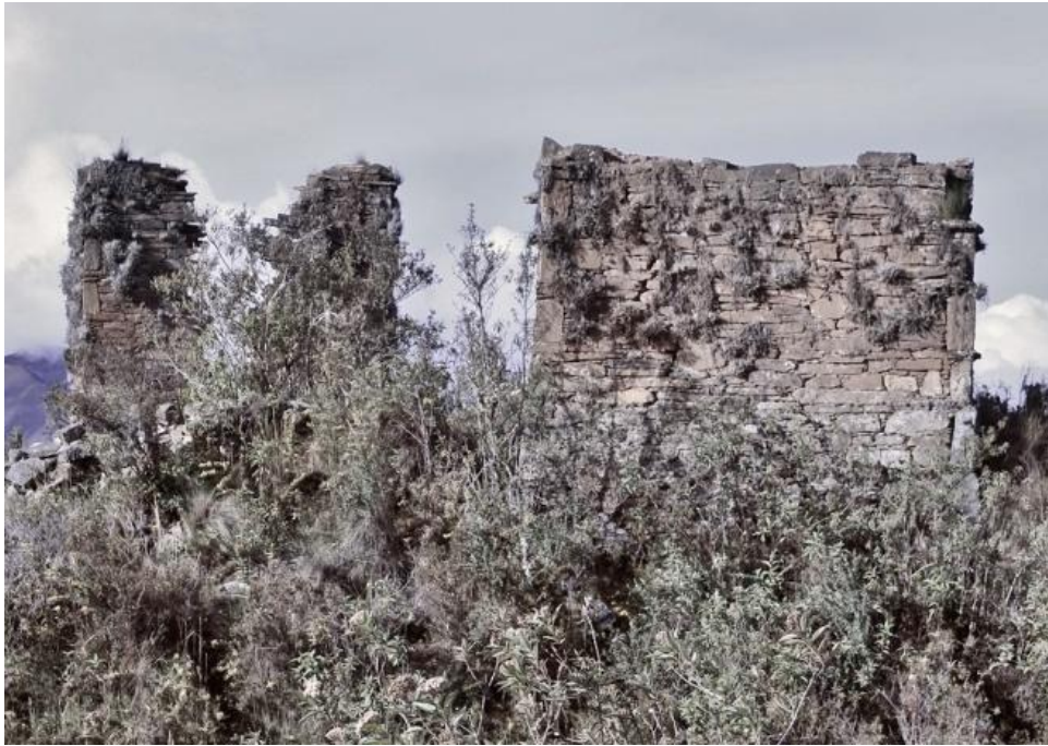
Tower (left) and headwall exterior (right)
