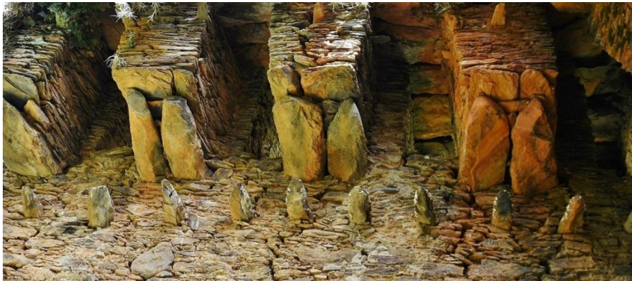
Corbels along the side wall
