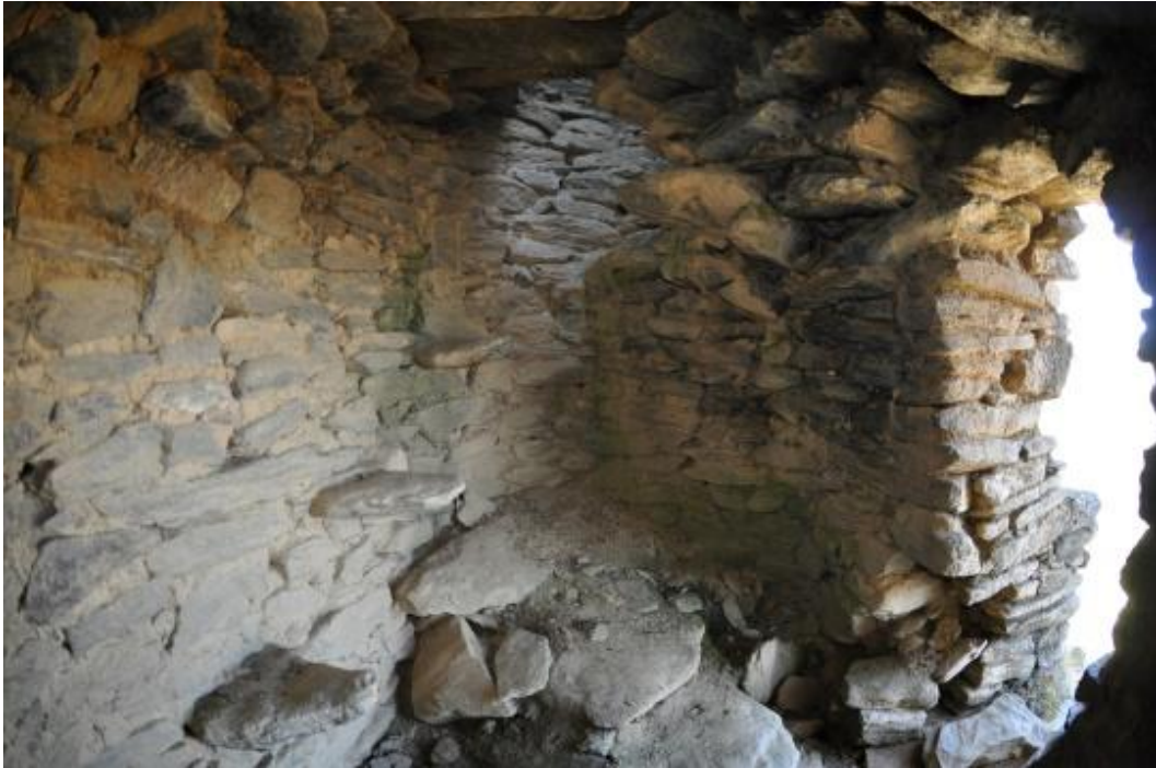
Chamber and access to the next storey in the headwall
