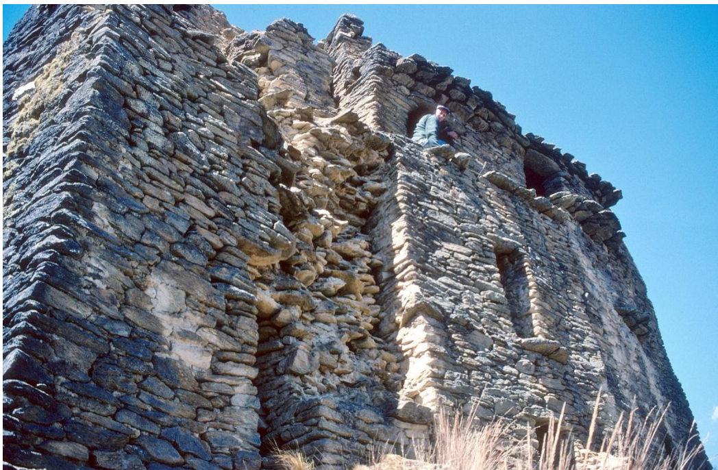
Interior side of the headwall (1996)
