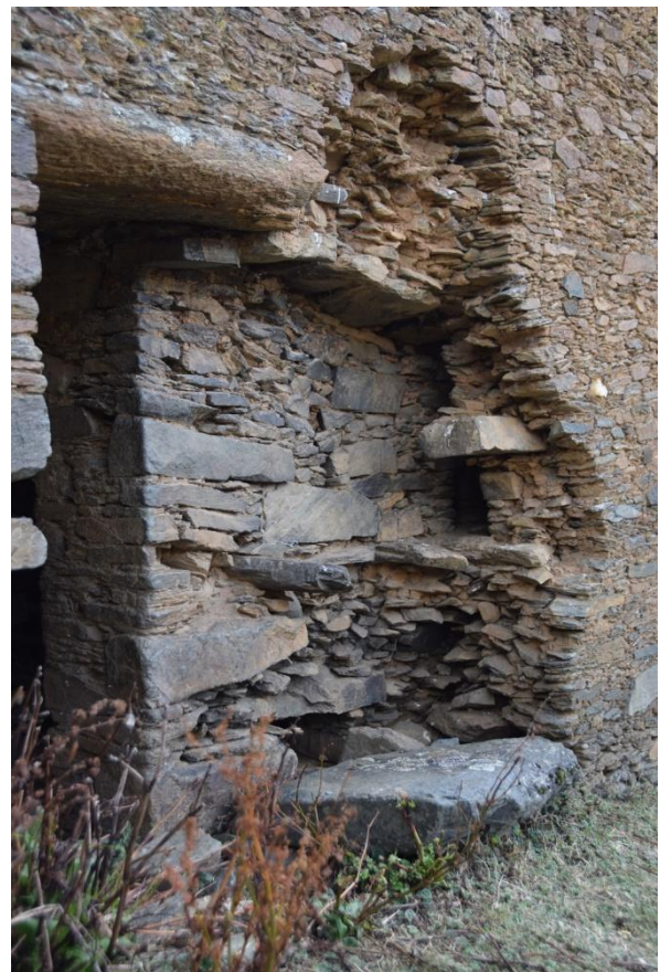
Detail of the double wall construction of a doorway jamb, common in torreones
