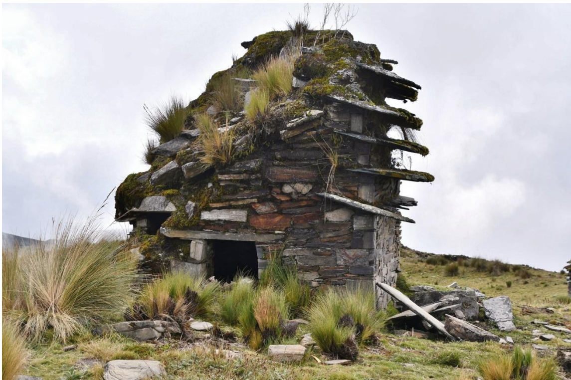
This is charnel house No. 3
