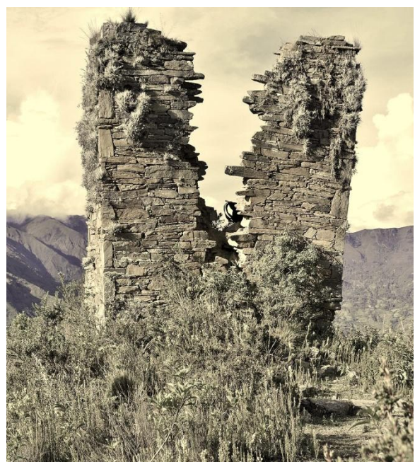
The tower is clearly ready to collapse
