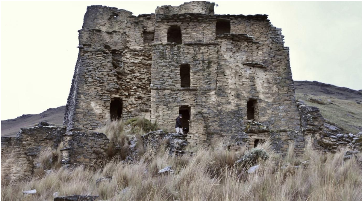
Interior side of the headwall
