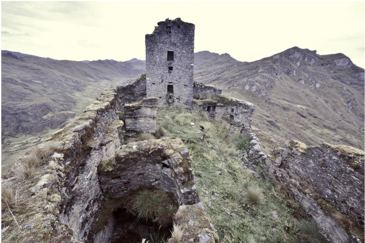
The headwall, seen from the tower over the entrance passage
