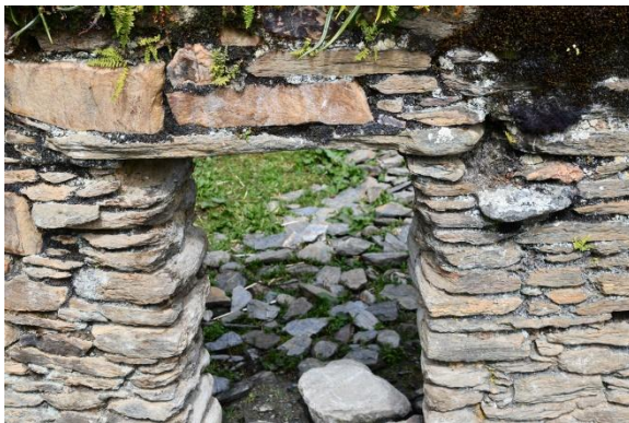
Outside and inside views of the doorway to the courtyard behind the round, conical tower. Note the pierced stones, presumably for anchoring some sort of door .
