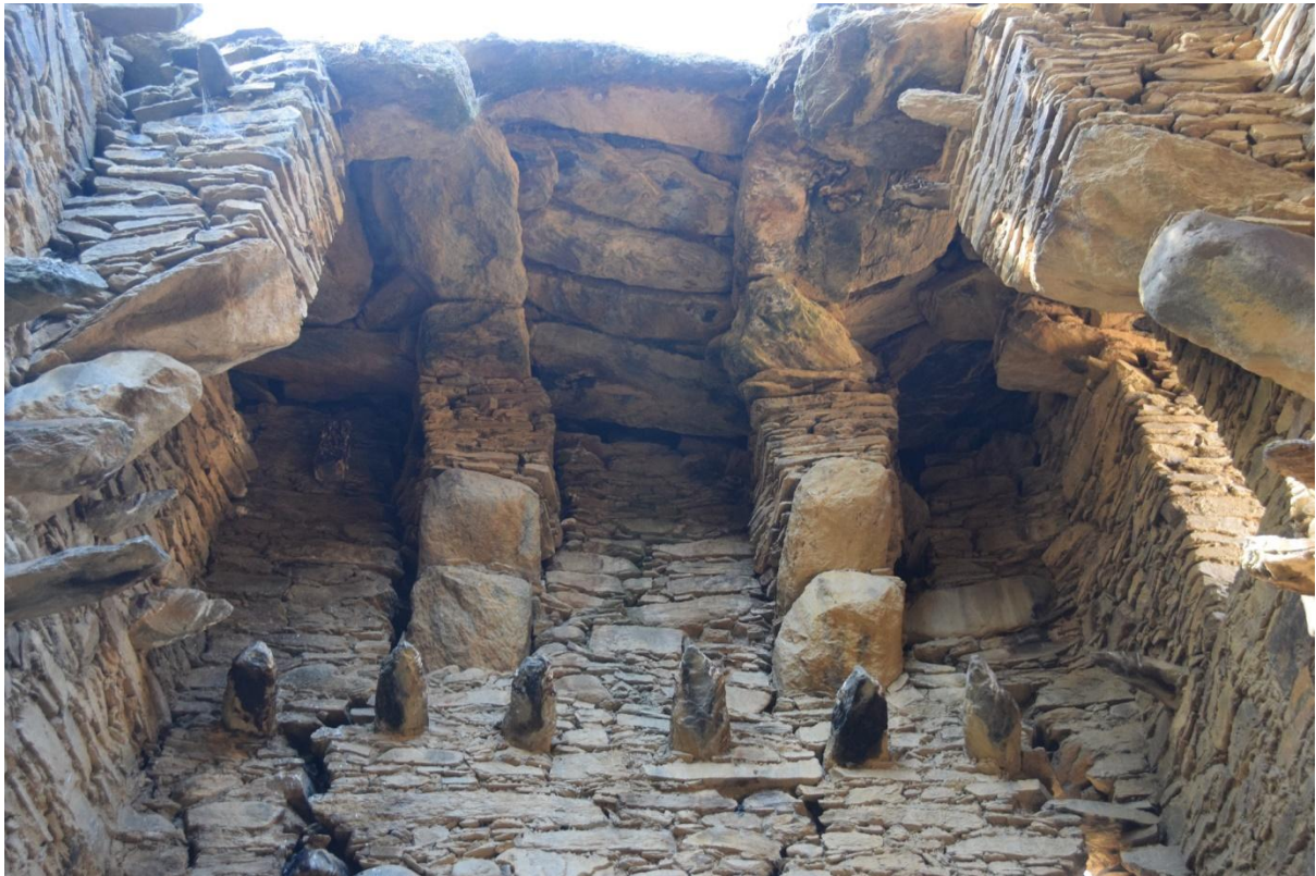
Detail of the corbel vaulting of the torreón
