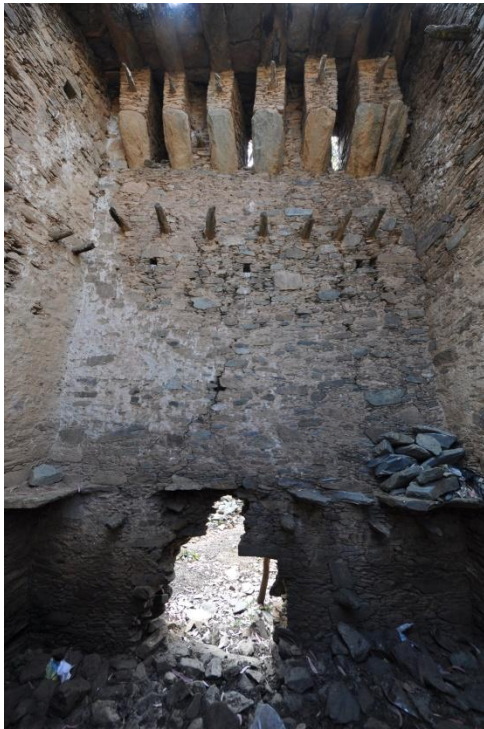
Detail of the corbels that supported the original vault of a torreón
