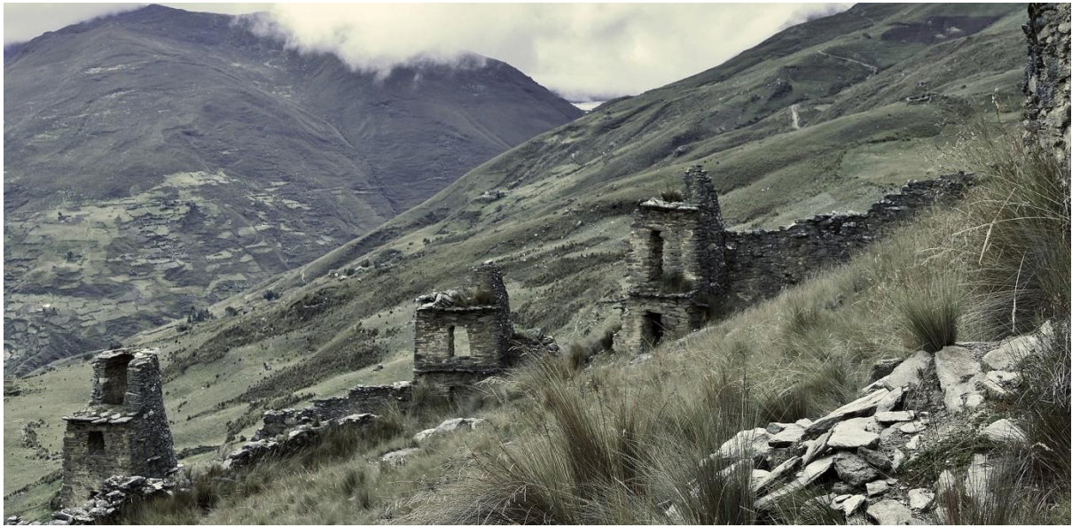
Curtain wall and towers – north side
