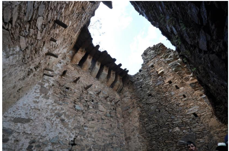
Detail of the corbels that supported the original vault of a torreón
