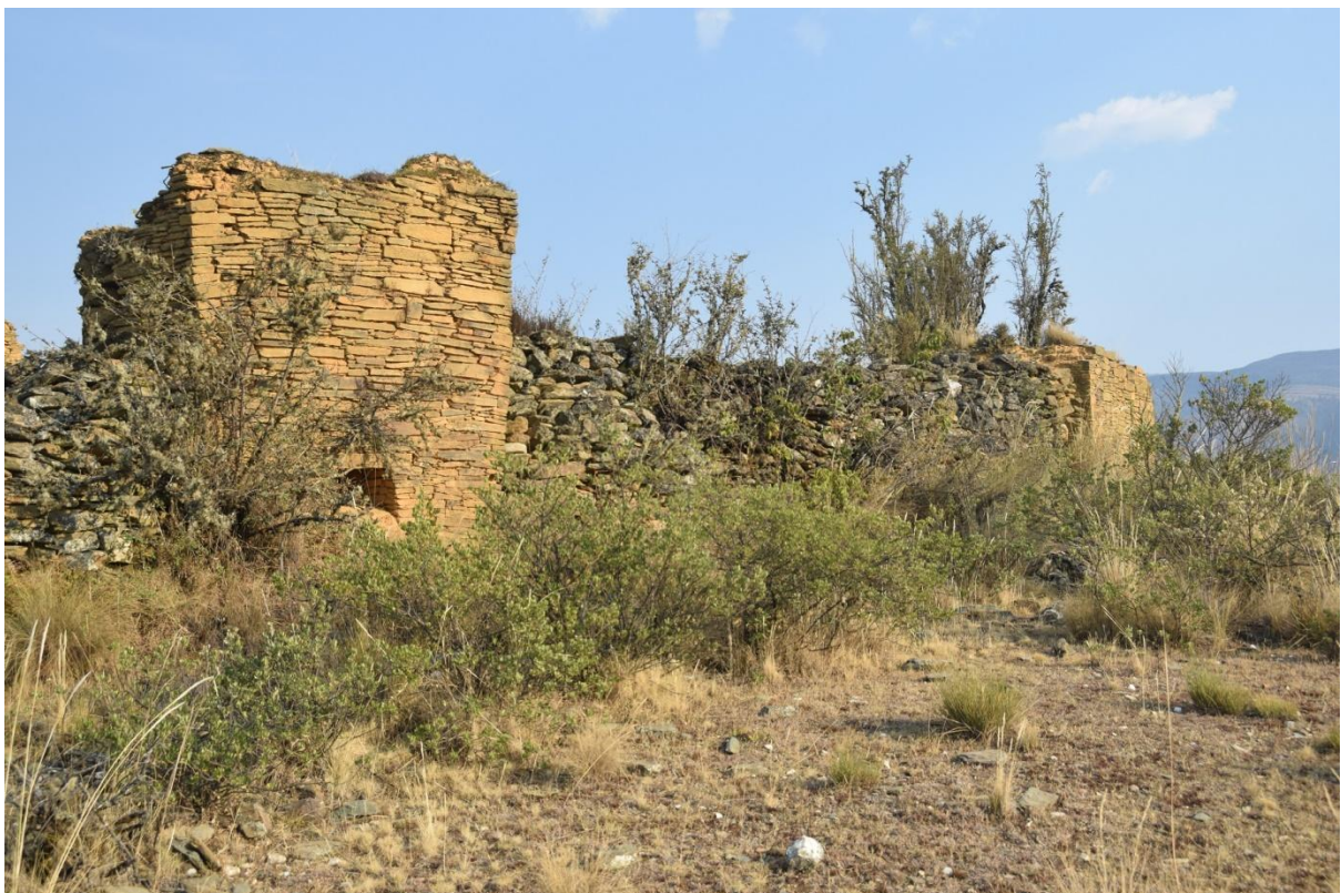
Outer perimeter wall facing down slope. This consists of original square towers and a later infill of stones presumably by campesinos (farmers) to make the site secure from livestock.
