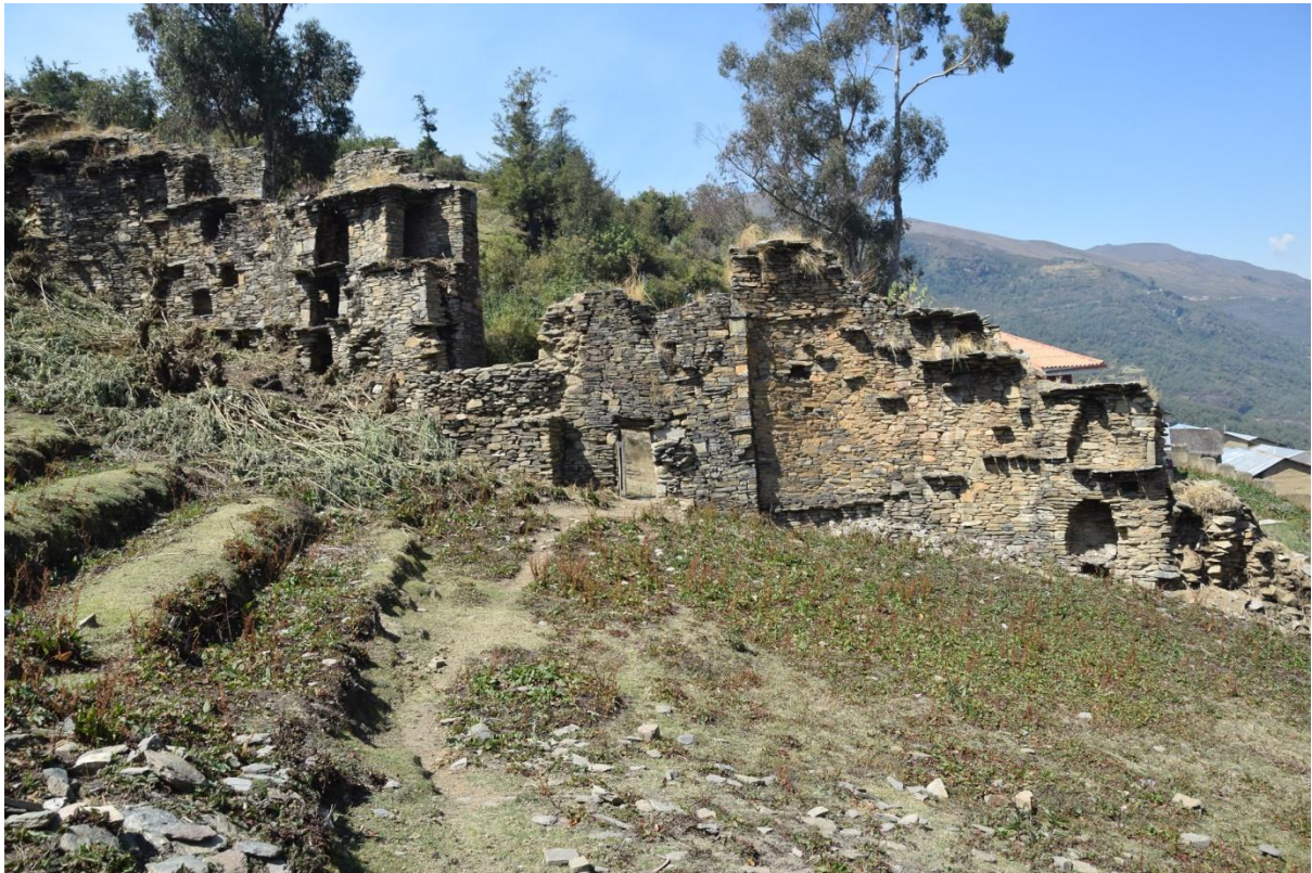
Interior of the curtain wall south of the headwall
