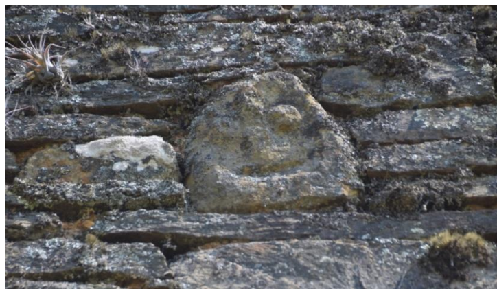
Relief of a face on the exterior of the headwall
