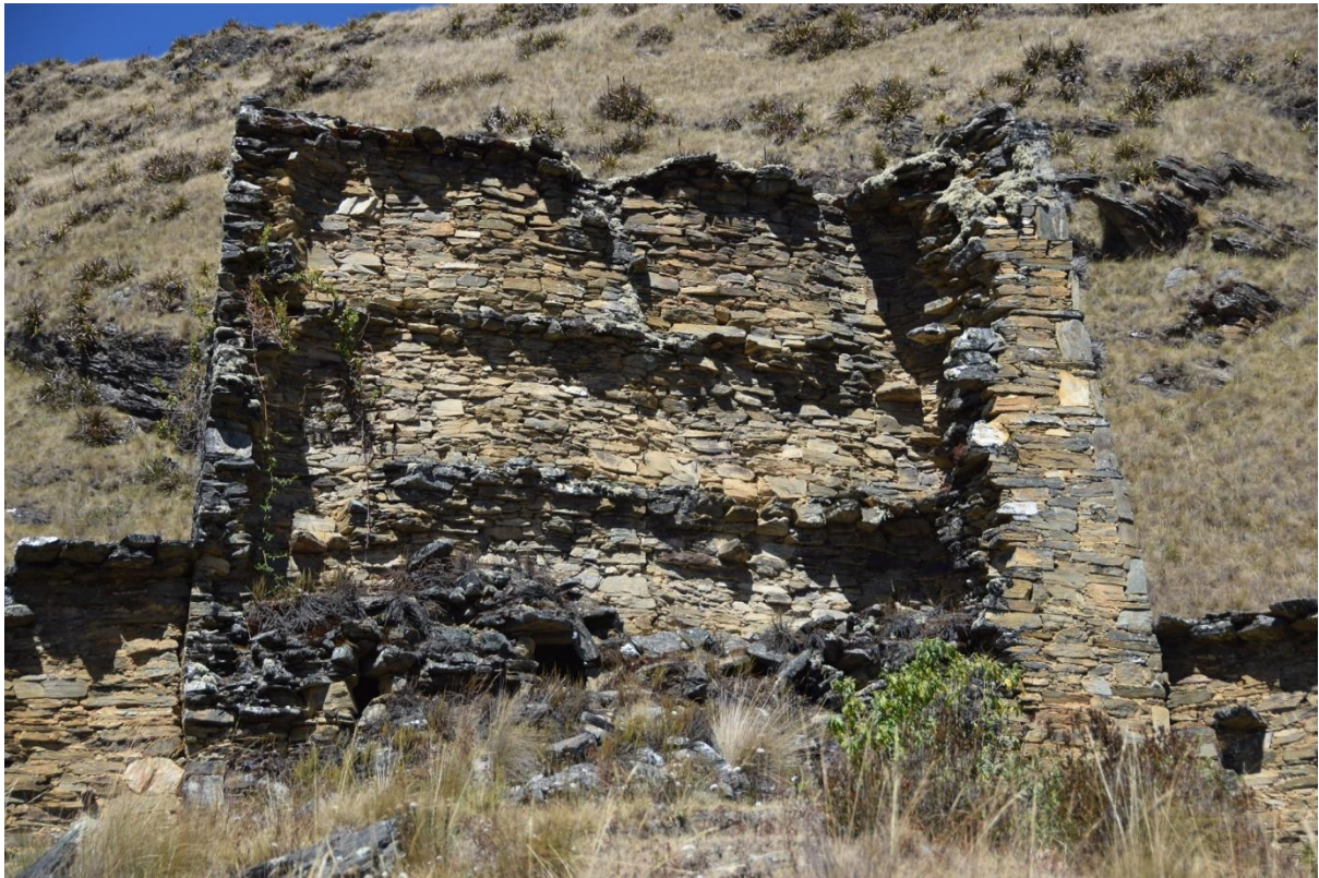
Detail of the headwall interior. Note how all the vaulted galleries have collapsed.
